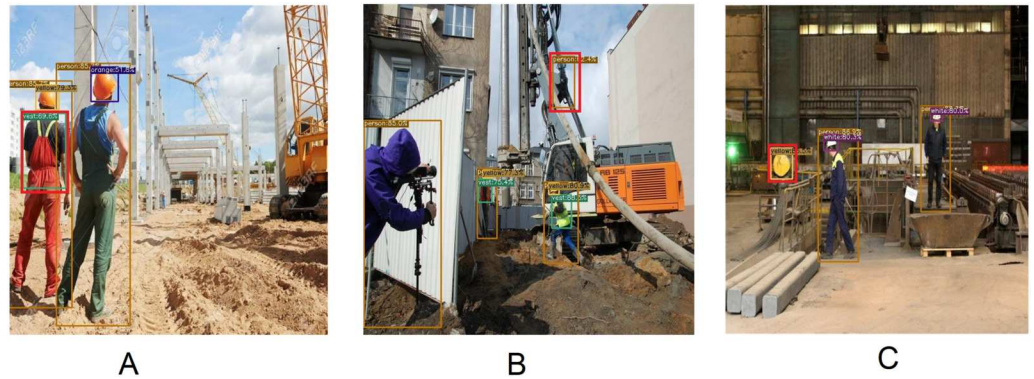
Figure 13 Incorrect detection of YOLOX-m architecture. (A) Something is detected as a vest which is not a vest. (B) An object is detected as a person which is not a person object. (C) A yellow color part of a machine is detected as a yellow hardhat.
