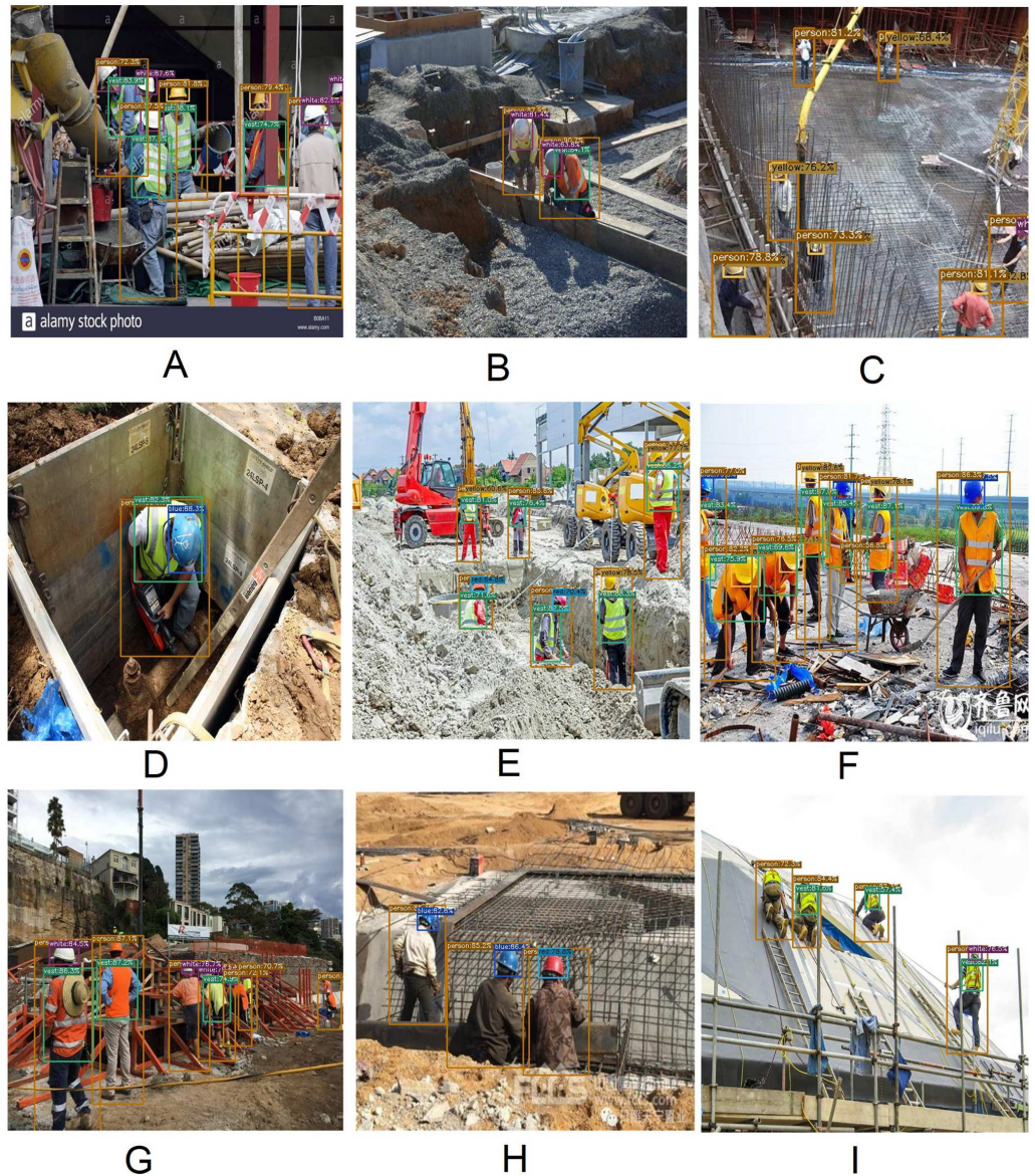
Figure 12 Satisfactory result of YOLOX-m architecture. (A) Objects are in dense condition. (B, C, H) Objects are small. (D, E, F, I) Objects are in natural working conditions.
