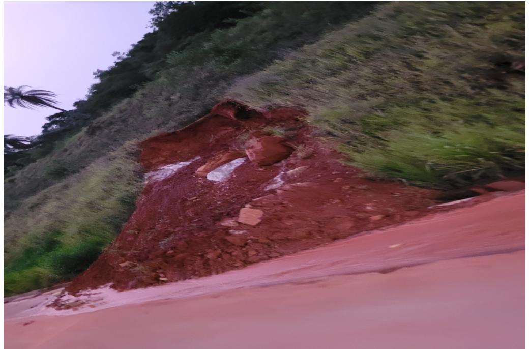
Figure 1 Landslide near Highway 381, Brazil 2022.
