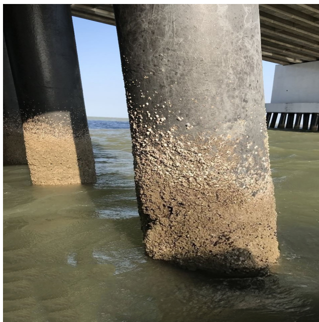
Figure 2 Appearance of pillars showing substrate attachment of barnacles.
