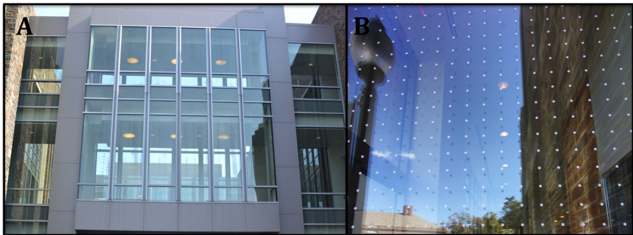
Figure 5. Bird deterrence dotted patterns on windows of Fitzpatrick building at Duke University. A: Glass passageways. B: Close up of dotted pattern. Photos: Casey Collins.
